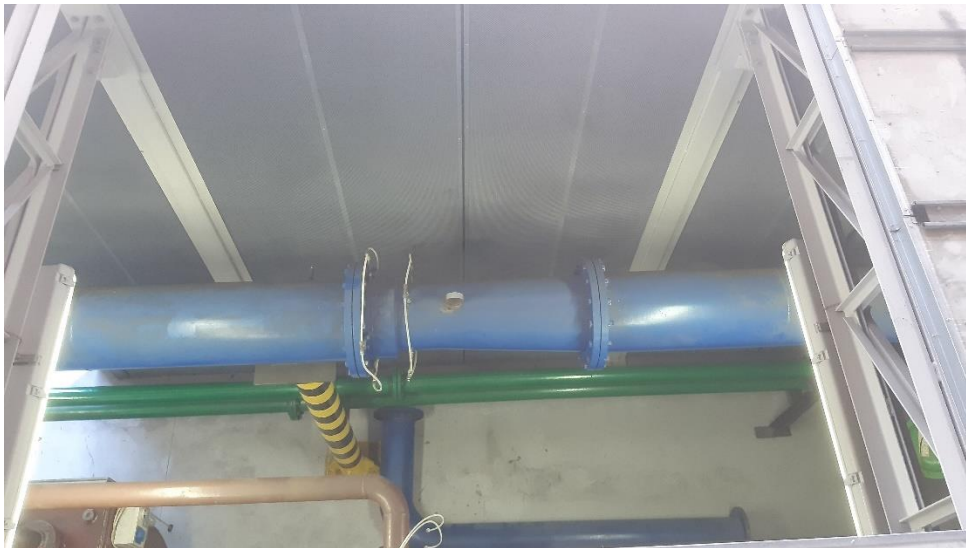
Figure 26 - Non standard classical venturi tube
