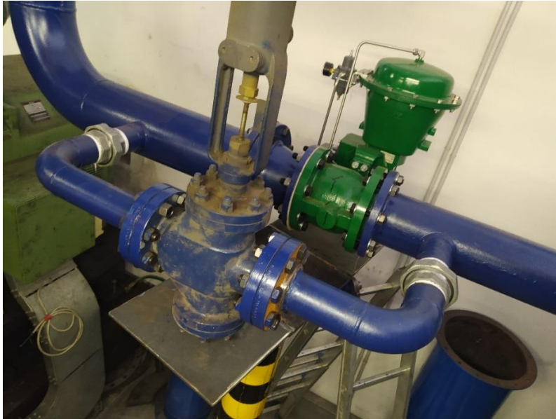
Figure 24 - Valves in parallel
