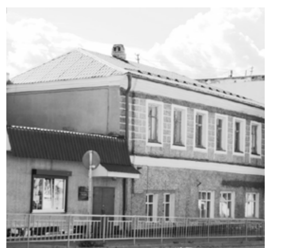
The building of Kimry Local Museum
