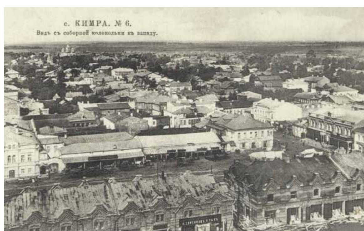
Construction of the Merchant Rows building, 1909, postcard
