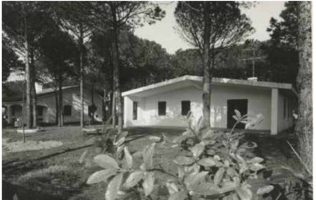
FIGURE 098: PHOTOGRAPHIC OFFICE MONTECATINI 1957/85
