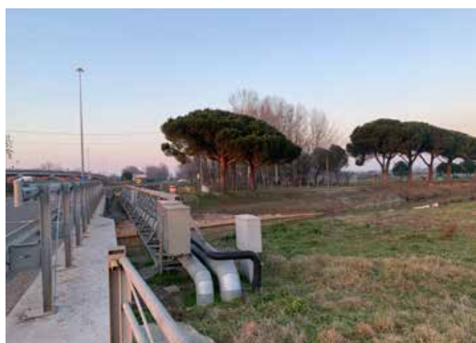
FIGURE 053: VIA ROMEA NORD, CANALI MAGNI, RAVENNA, JANUARY 2022
