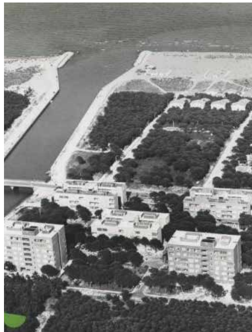
FIGURE 096: PHOTOGRAPHIC OFFICE MONTECATINI 1957/85
