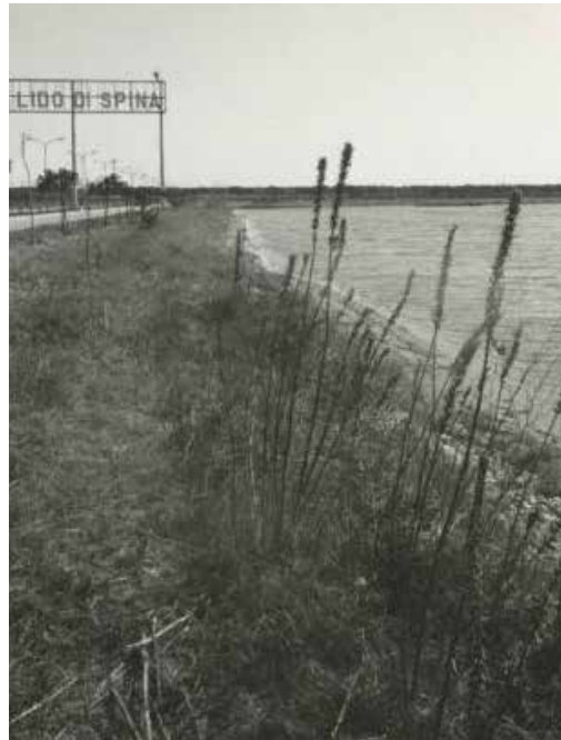
FIGURE 094: PHOTOGRAPHIC OFFICE MONTECATINI 1957/85
