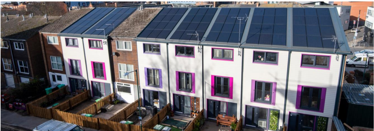
Figure 14 Nottingham single family houses after a Energiesprong renovation
