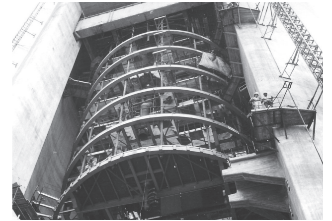
Fig. 24. Construction of the chimneys (1971)
