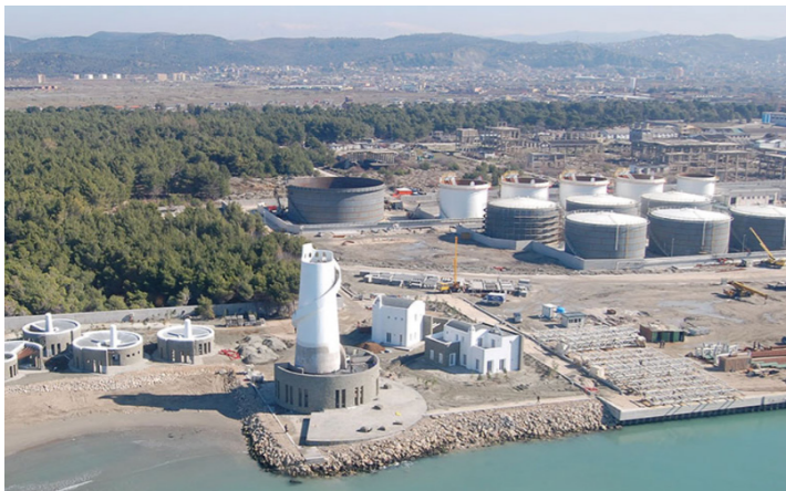
Figure 117 - La Petrolifera Italo Albanese Sh.A. (PIA) operates a coastal terminal for LPG, Oil, its by products and additional liquid and dry products in the Bay of Vlora. Its proximity to the sea, forest and city makes it a major pollutant and increased toxicity levels by the environmental report by Arpa Lombardia. The industrial zone located by the encroached forest poses a major potential risk and health hazard to the marine life and inhabitants of the city of Vlora. Proposing a project thus in the lower reach of the Soda forest is also a way to ensure that encroachment is reduced and protective measures taken. Photo by G&A Projekt.
