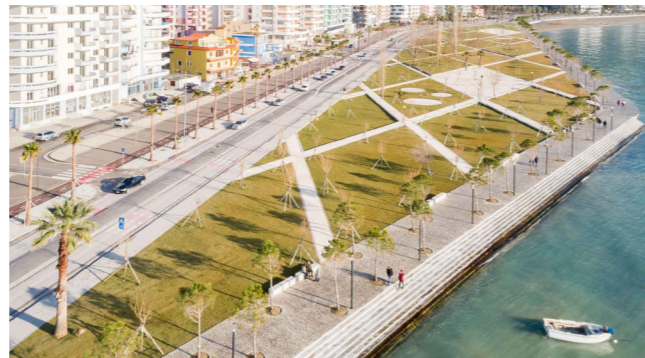
Figure 127 - F Aerial view of the park with its reticular geometry of white paths.
