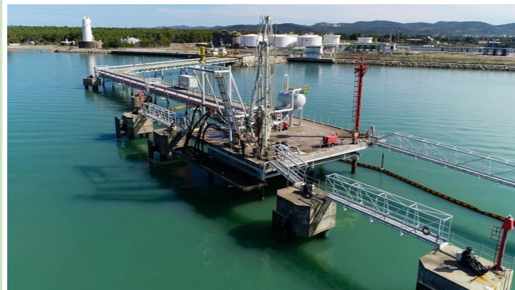
Figure 105 - The port access to the petroleum depot.
