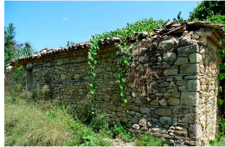
Figure 21 - Remains of a traditional dwelling in the hill quarter with horizontal reinforcing timber elements. (Author)
