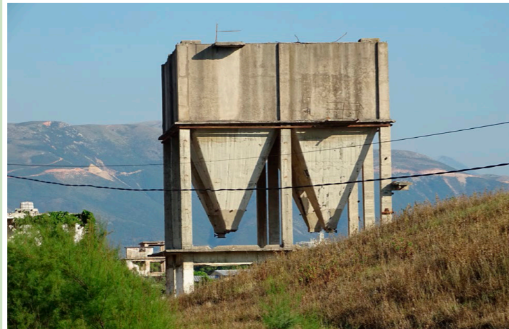
Figure 103 - Remnants of Uzina PVC plant.
