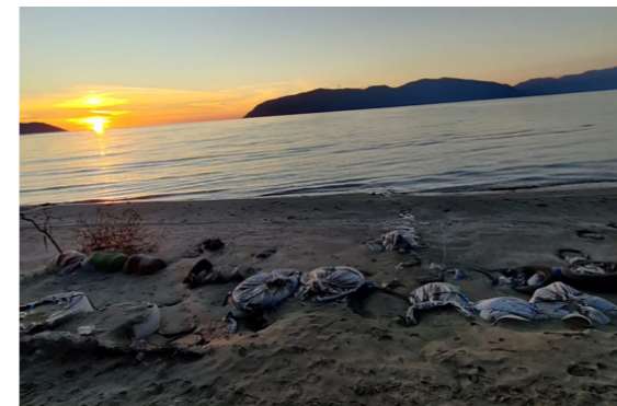
Figure 110 - Failed erosion measures at the beach, Soda forest. (Author)
