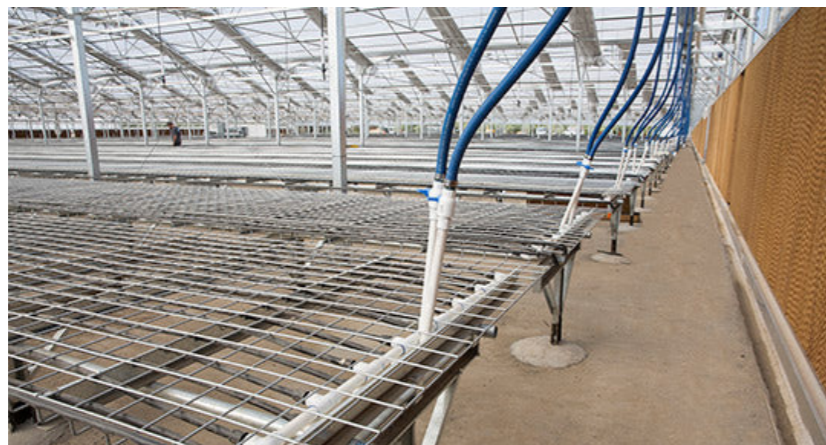
Picture of U.B.H.I. (Under bench heating integration) system.
