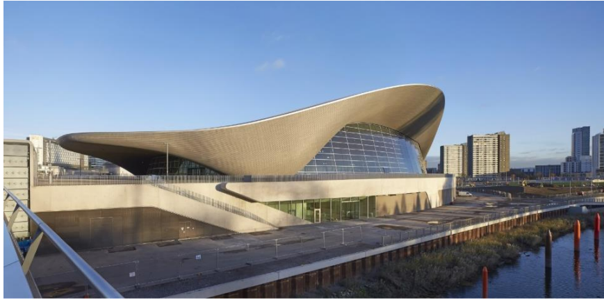
Image 5.6 - Exterior view of the London Aquatics Centre. Source: Archello.
