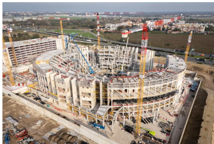
Image 4.2 - Construction phase of Unipol Dome in the Milano Santa Giulia redevelopment area. Source: The Plan
