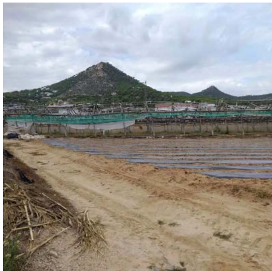
Path between the greenhouses and fields of Vilassar de Mar Problem: Path in decay; instable path; lack of safety; abandoned fields and greenhouses Potentiality: Connecting element of the landscape; reuse of agricultural spaces in the park
