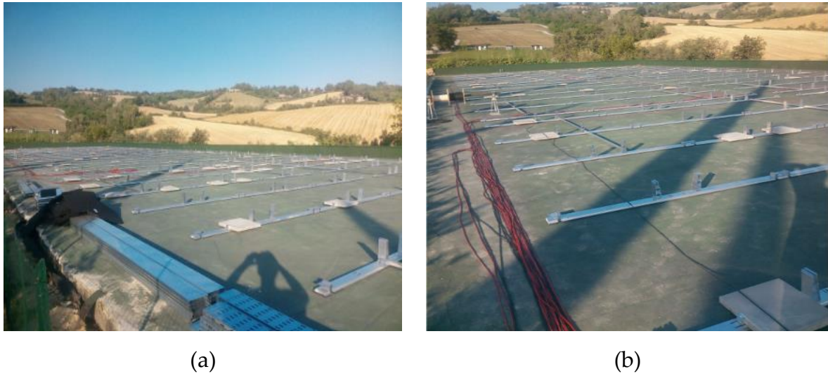
Figura 65: (a) Substructures installation, (b) DC cable installation
