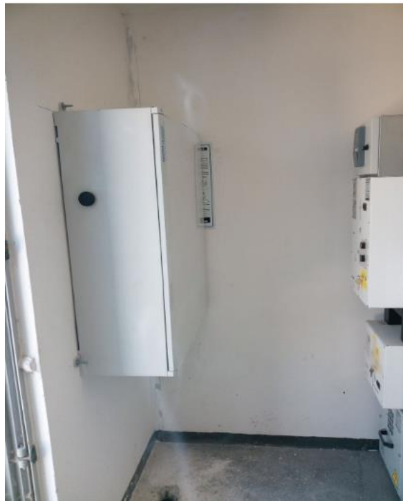
Figura 64: Interface board installation
