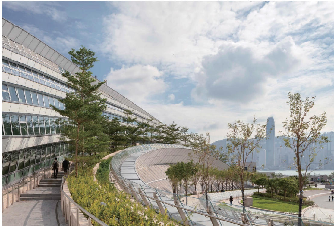
Figure 4.3.3.3.a - Pedestrian ramp on roof connecting to the ground floor © Paul Warchol
