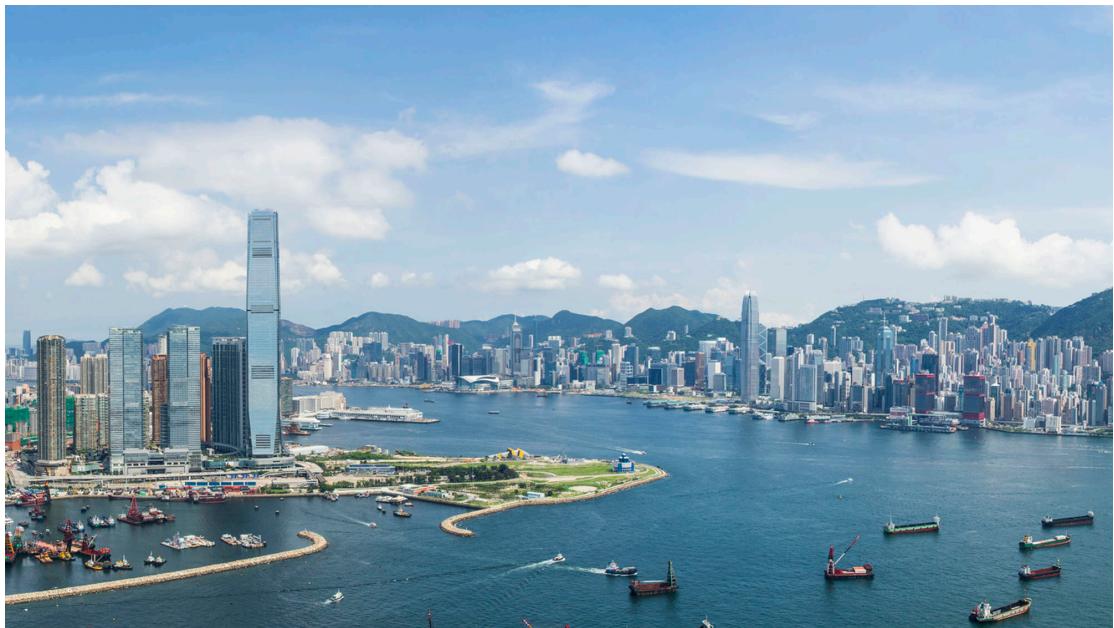
Figure 4.3.8.c - ICC and International Finance Centre on the opposite shore have formed a stunning gateway across the Victoria Harbour. (Source: https://www.arup.com/projects/international-commerce-center-hong-kong )
