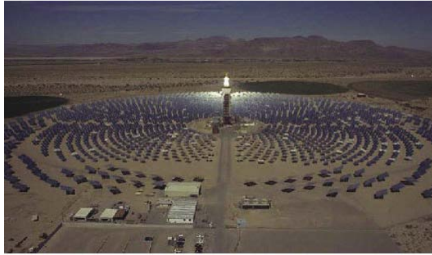
Figure 1.14: Circular heliostat field of "Solar Two" plant
