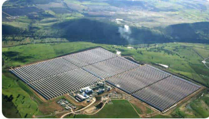
Figure 1.19: Planta solar Puertollano, Spain
