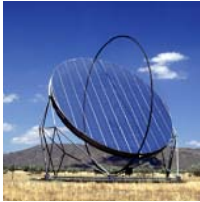
Figure 3.19: ASM-150 stretched membrane heliostat
