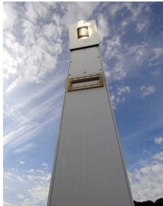
Figure 4.9: The Jülich plant tower
