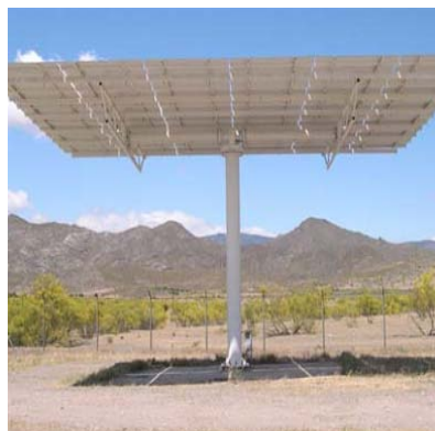
Figure 3.21: Example of heliostat pedestal.
