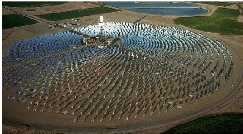
Figure 3.23: Solar One power plant
