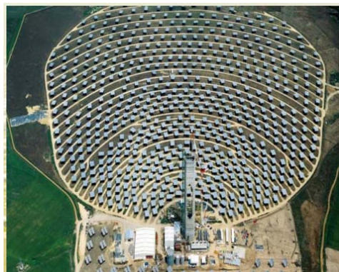
Figure 3.26: PS10 solar field
