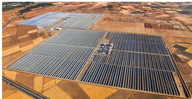
Figure 1.10: Andasol I and II parabolic trough power plants
