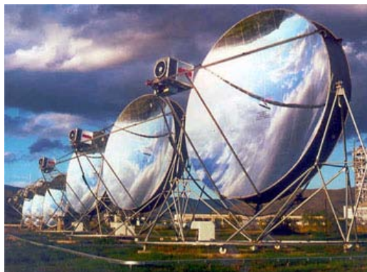
Figure 1.12: Parabolic dishes with Stirling engine
