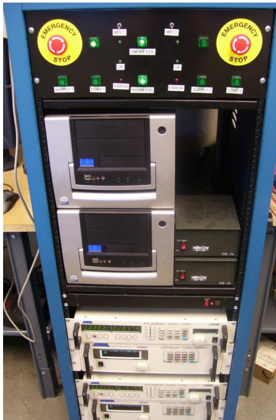
Figure 5.16. Battery test bench.
