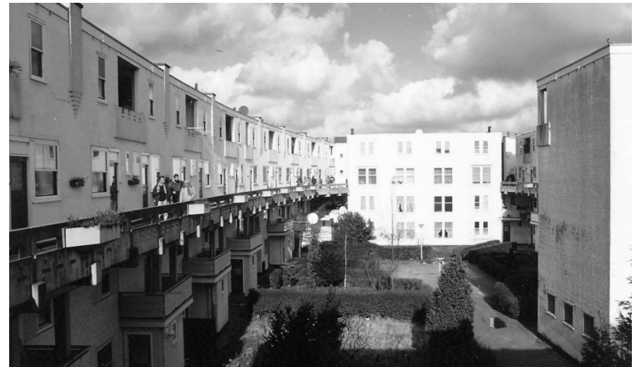
Figure 54. Spangen after the renovation, Michiel Brinkman, Rotterdam (1919-22) (author's figure, 2008).
