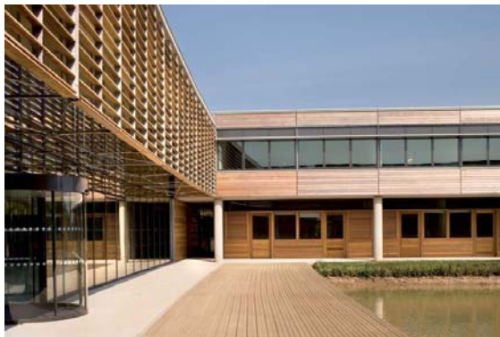
- Hopkins, Butterfield Park Innovation Centre, Luton (UK), 2007
