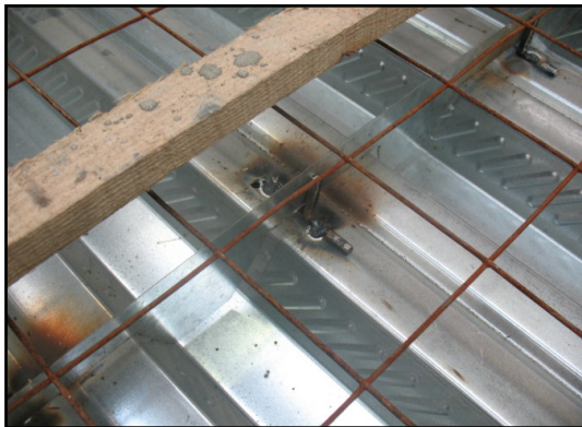
Figure 38 - Crack inducer detail
