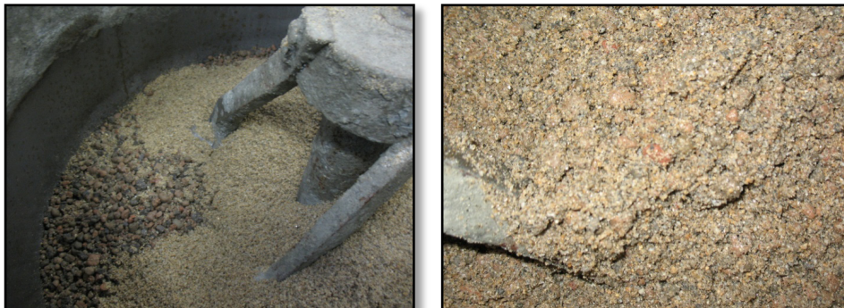
Figure 8 - Concrete mixing first phase
