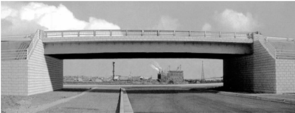
Figura 1.11: Nishihama Bridge ( Nakamura, 2002 )
