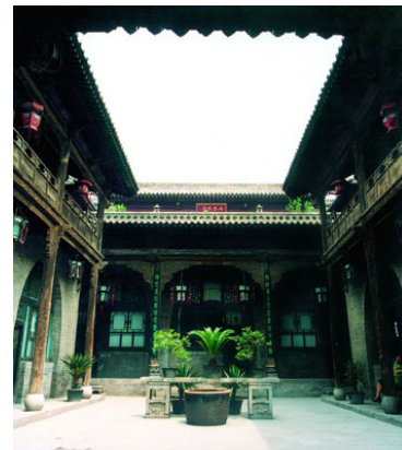
Figure 51: Courtyard is smaller in the hot summer and cold winter climate zone (middle of China) to prevent overheating in summer
