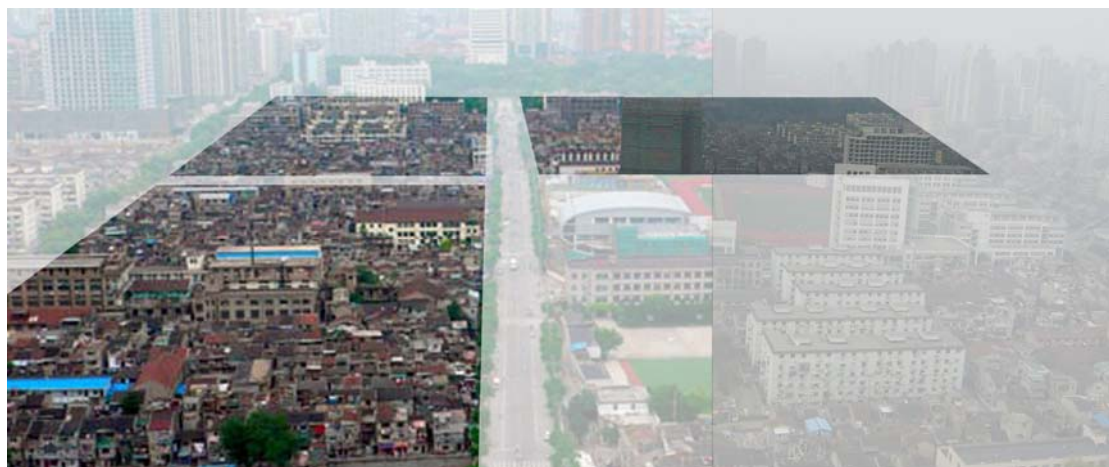
Figure 26: The bird view of project site (Heping Park on the north and Sport Center on the east)
