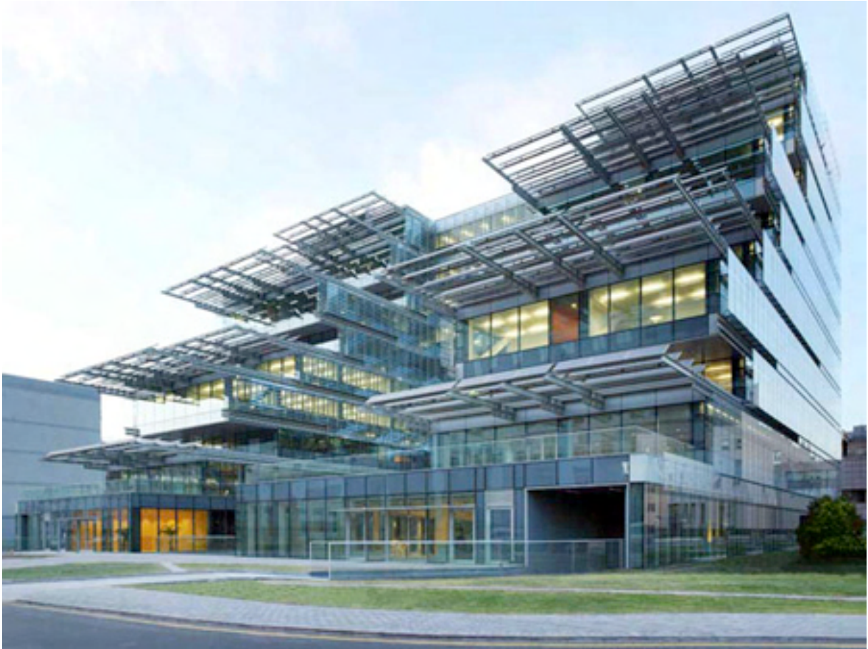
Figura 15 - SIEEB: Sino-Italian Ecological and Energy Efficient Building di M. Cucinella, 2003 - fonte Green.mnp
