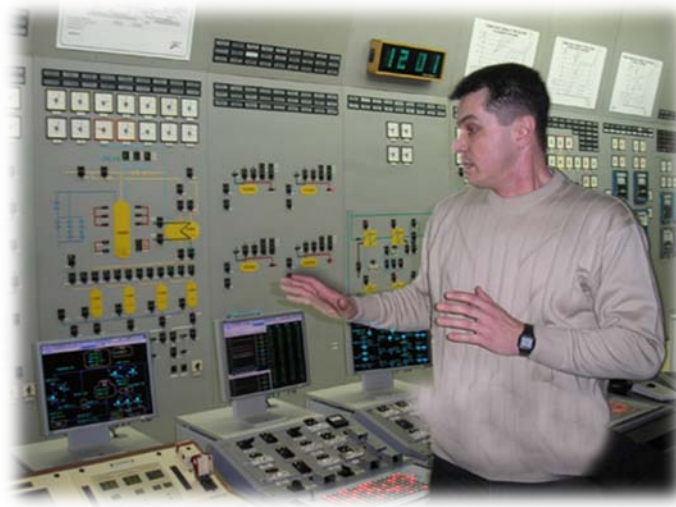
Image. Training center of Zaporizhzhya NPP. Energoatom. 2009
