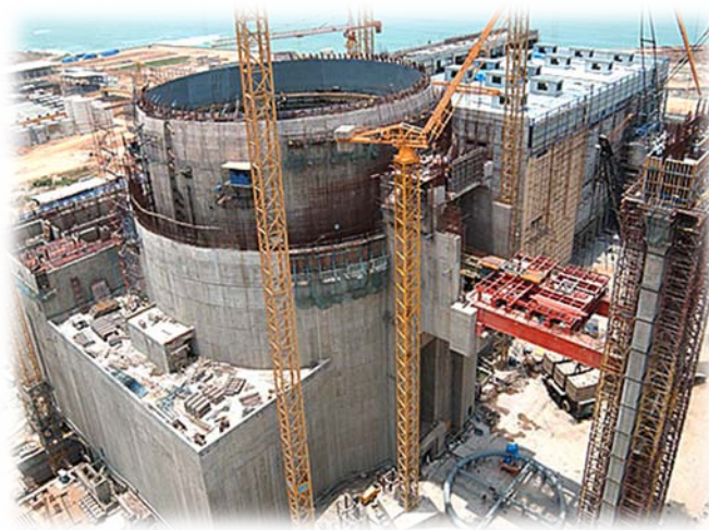
Image. NPP construction. Consulting center. 2010
