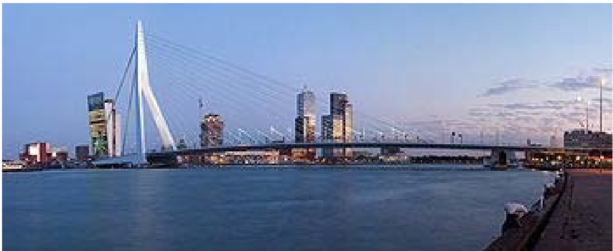
Fig. 1.5 Erasmus Bridge Rotterdam
