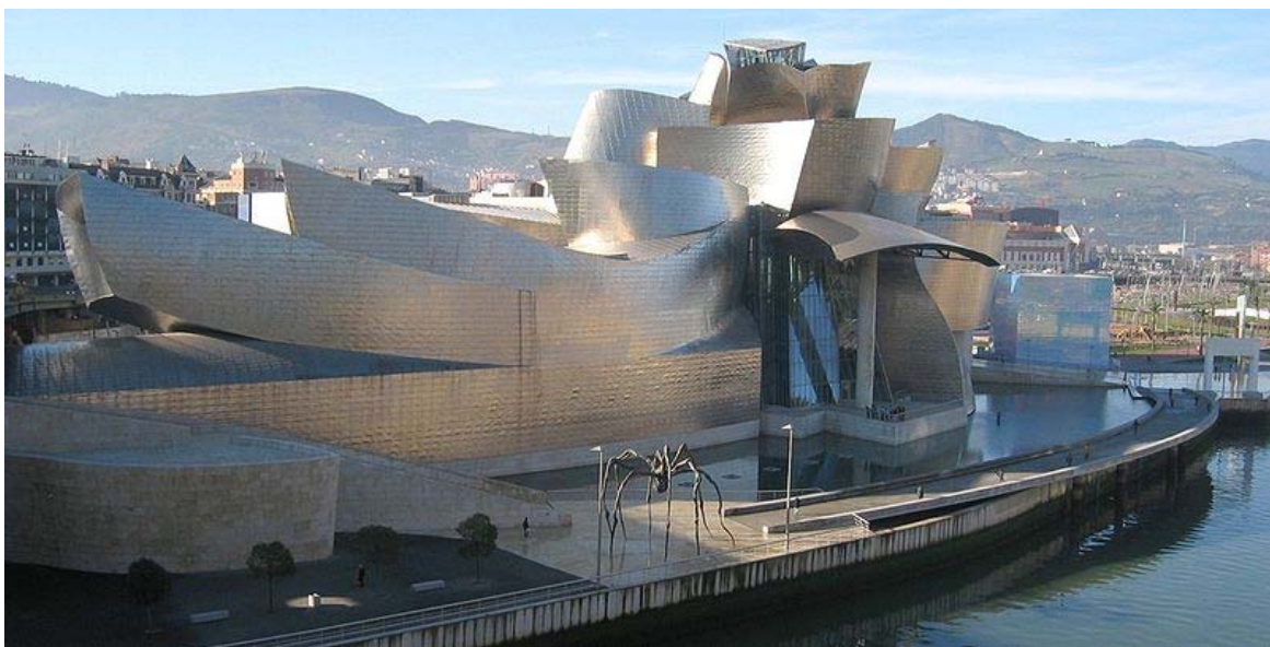
Fig.1.16. The Guggenheim Museum Bilbao was the first buildings in Europe and to be sheathed in titanium panels.
