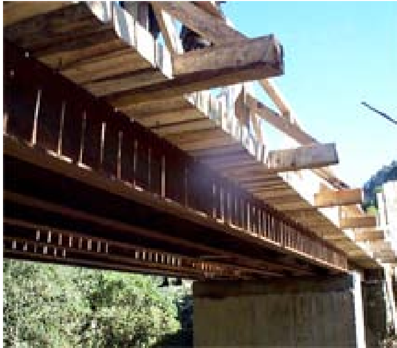
Fig.1.14. U.S. Army maintains vanadium microalloyed steel bridge designs for rapid reconstruction during deployed operations.
