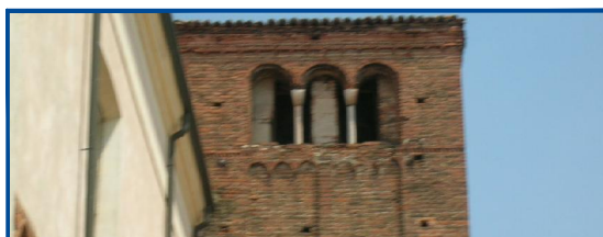
107. Cella campanaria a trifora
