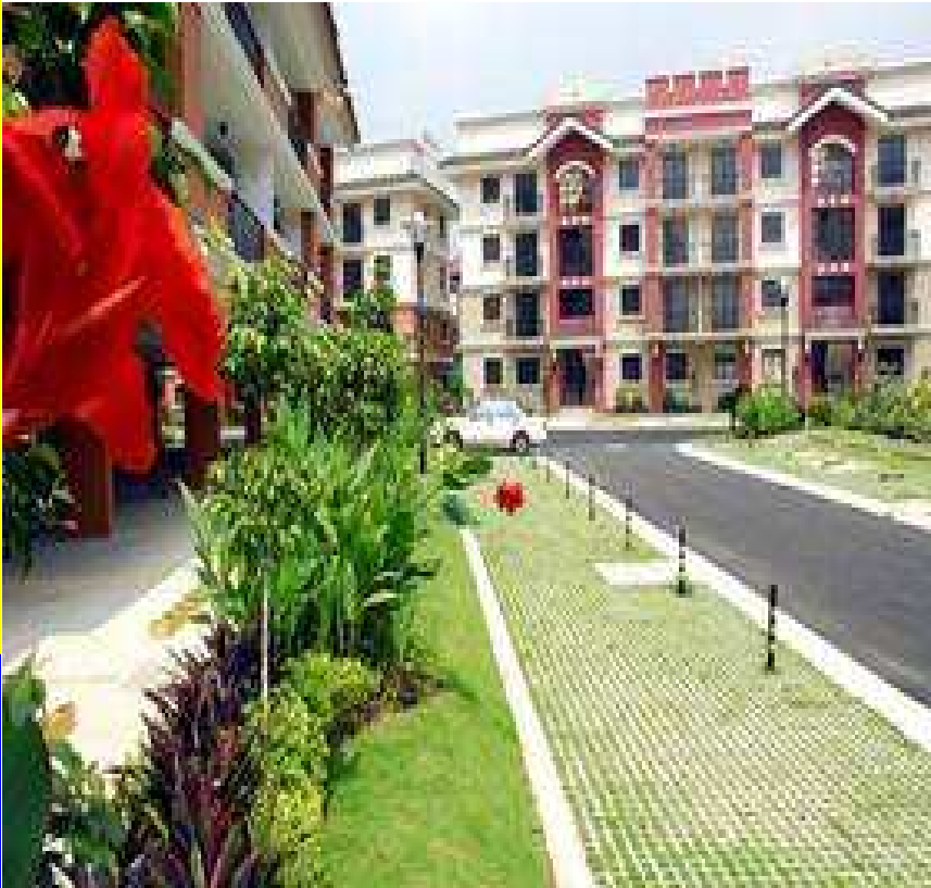
Fig.7. Above left: Student hostel facilities,
