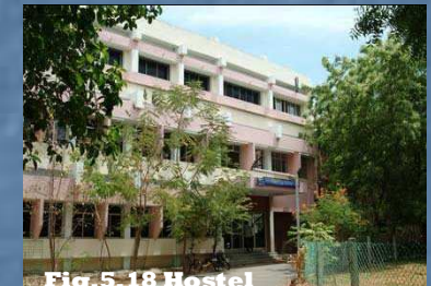
Fig. 5.18 Hostel buildings for women
