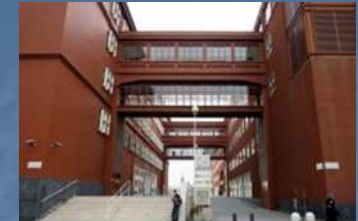
Fig.2.1 Pirelli buildings redone
