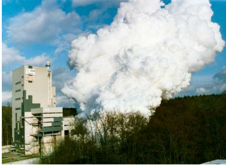
Figure C.1: P5 test facility at DLR Lampolshausen
