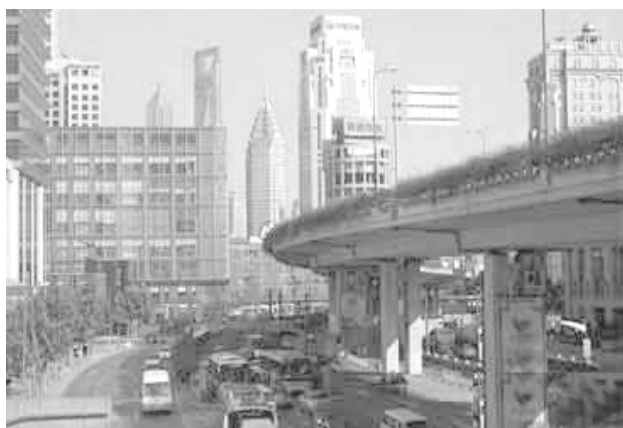
Photo of Shanghai Contemporary Transportation System
