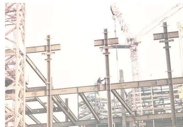
Photo of Construction Site in Shanghai
