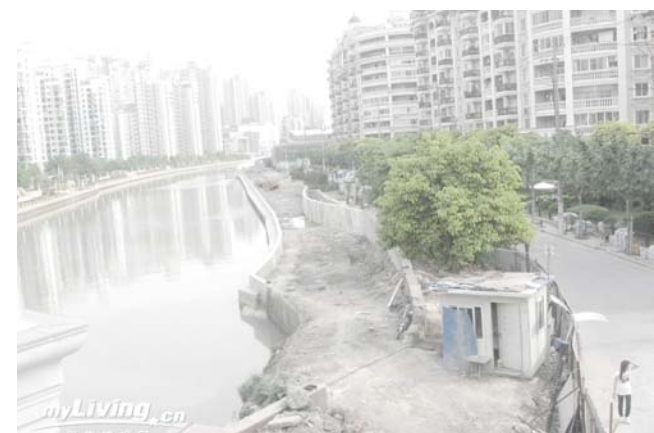
Photo of Flood Control Wall Along Suzhou Creek
