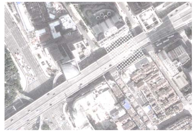
Satellite Map: The Sample Site, Part of Yan'An Viaduct
