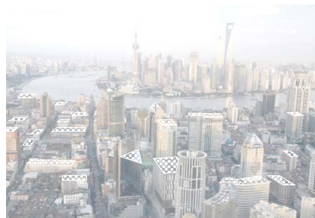
Photo: The Aerial View of Roofs of Shanghai City Center
