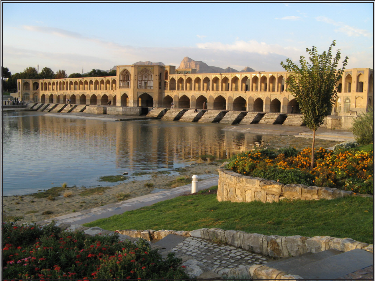
Ponte Khaju a Isfahan, 2009
