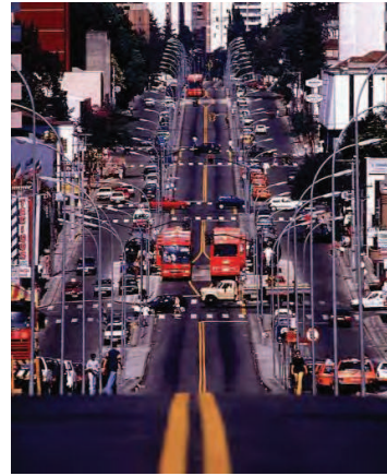
IMAGE 04: Structural Axis. The city is divided into structural axis, realized for the passage of the Bus Rapid Transport.
