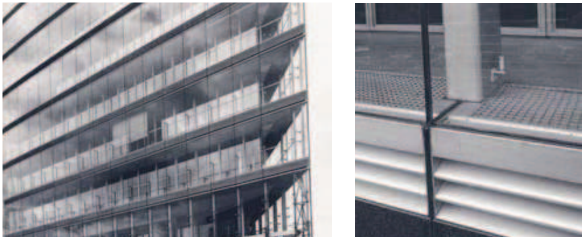
Images 32 and 33: Dusseldorf Stadttor building and its natural ventilation system.
