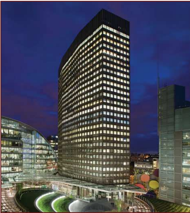
Figura 57: Portland House, Londra (1963)
