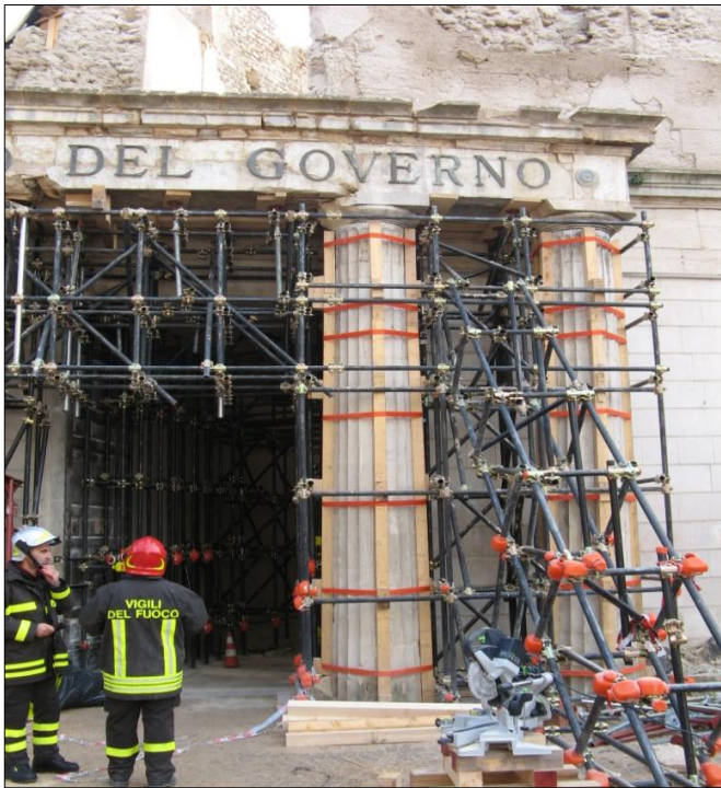
Figure 44 Examples of Steel Pipe Vertical Shoring Systems
