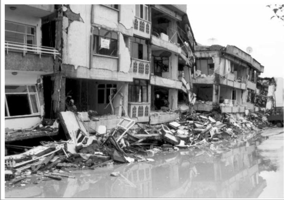
Figure 53 Soft storey failure in 1999 Kocaeli Earthquake
