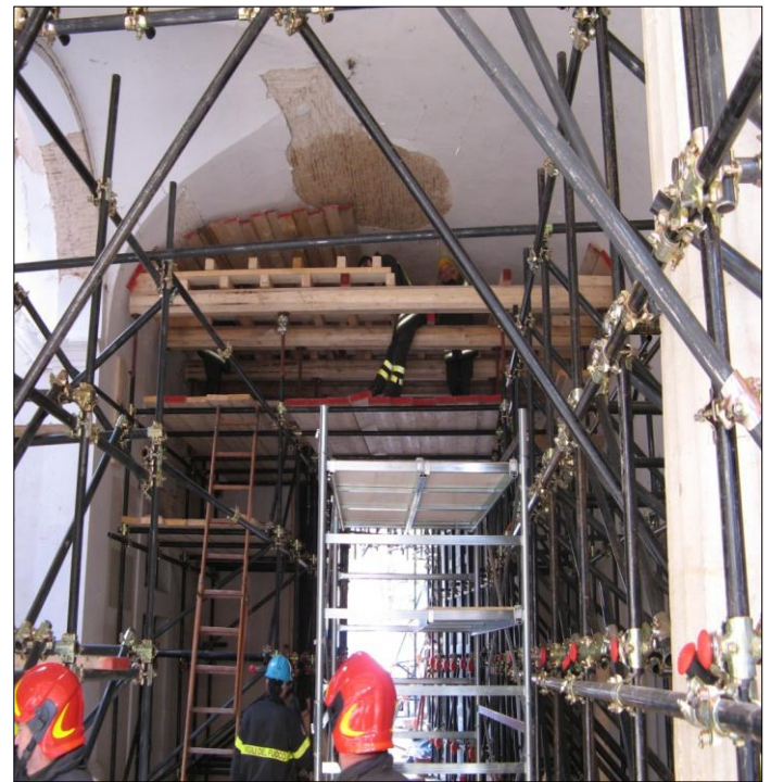
Figure 44 Examples of Steel Pipe Vertical Shoring Systems
