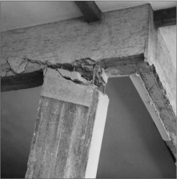
Figure 56 Examples of Poor Detailing Failure
