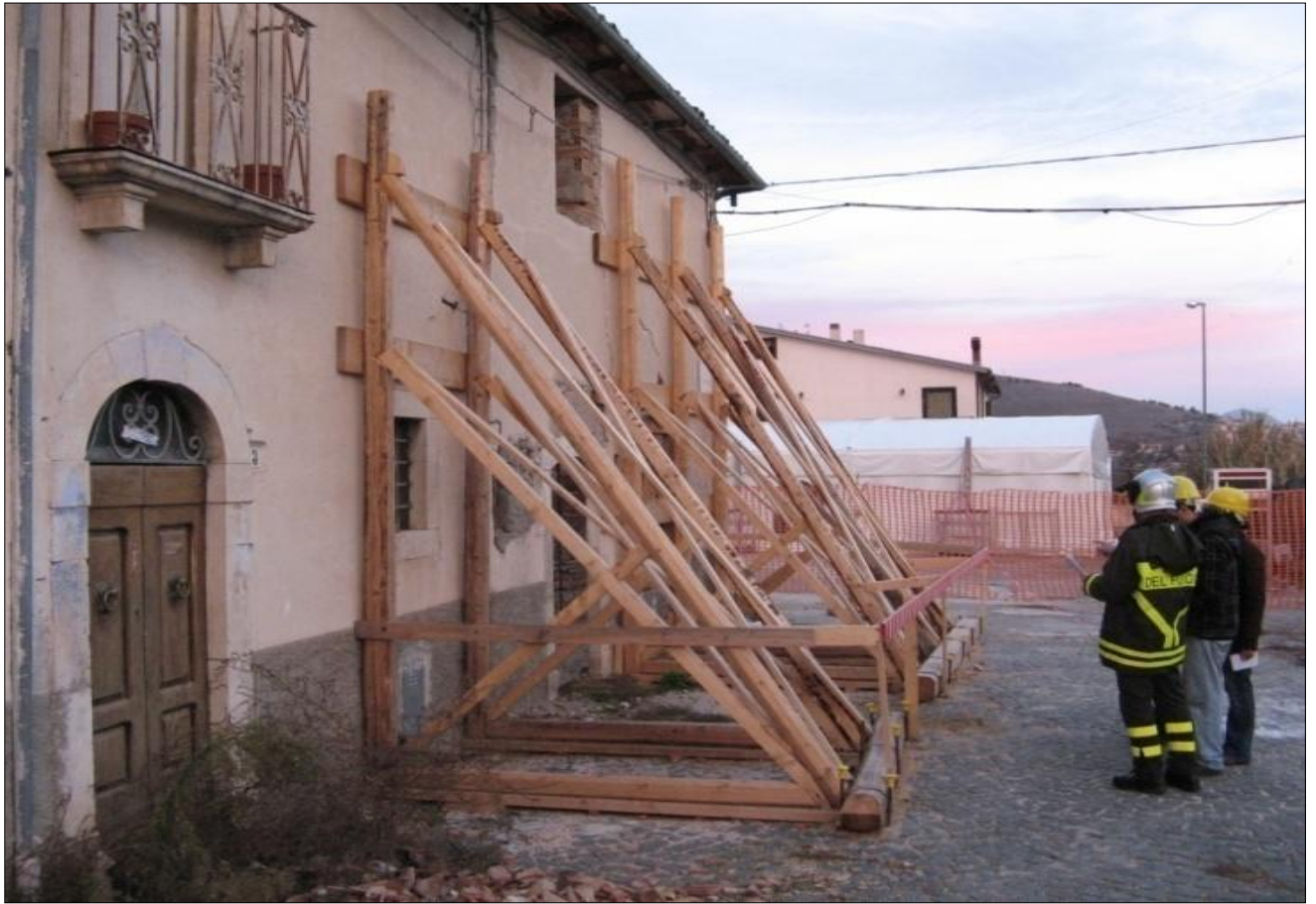
Figure 48 An application of shoring in L'Aquila
