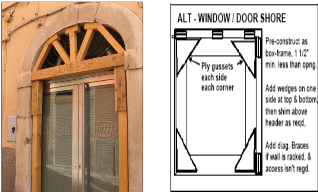
Figure 42 Window and door shores
