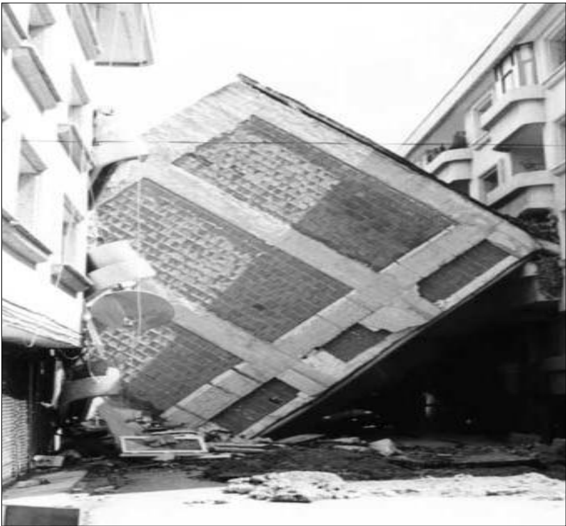
Figure 54 Soft Storey Failure in Kocaeli 1999
