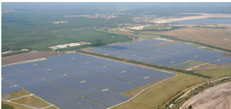
Figure 1.9: Finsterwalde Solar Park, Germany.
