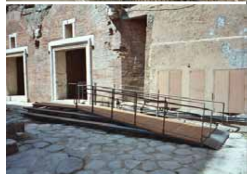
Figure 48/49/59/51/52: Mercati di Traiano restaurati
