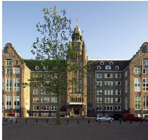
fig 1.13 Lloyd Hotel & Cultural Embassy, vista esterna; www.laterooms.com
