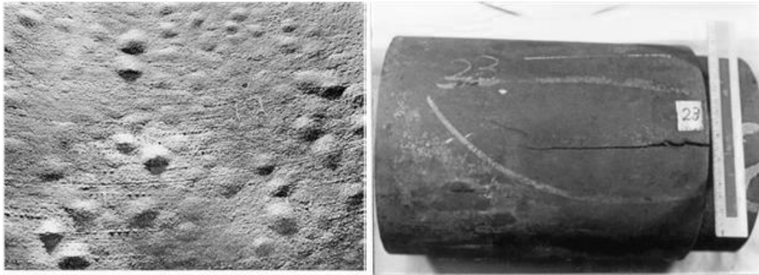
Figure 1.5: Hydrogen blisters on a pressure vessel [4] and HIC on a pipeline.
