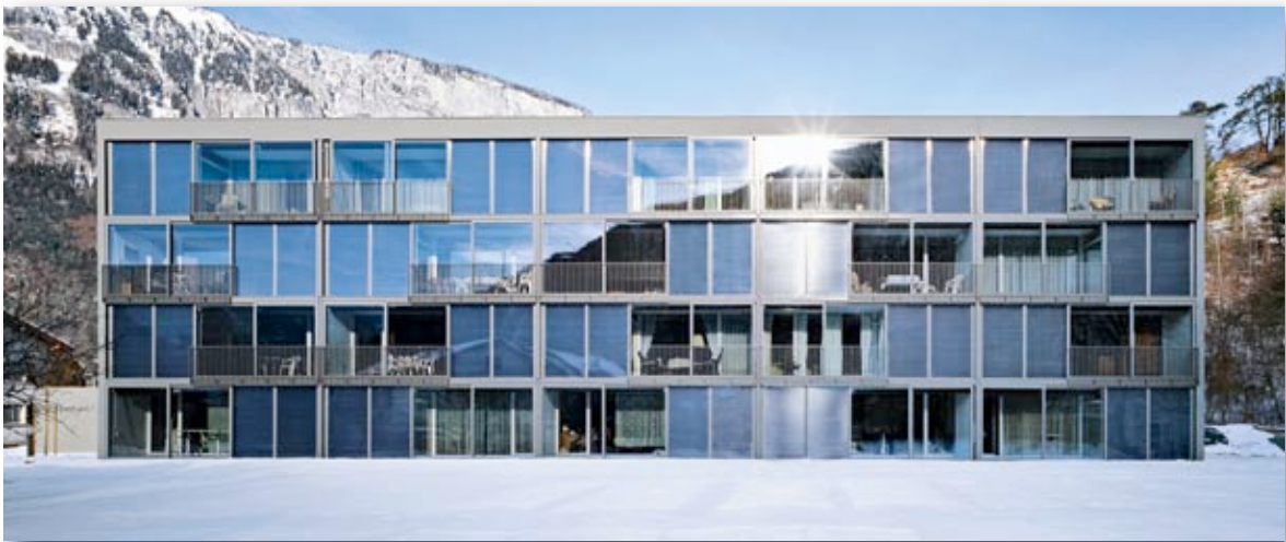
Image 14: Front facade of the home for the elderly in Ems
