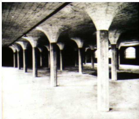
Fig.40. Maillart, pilastro a fungo (1908)
