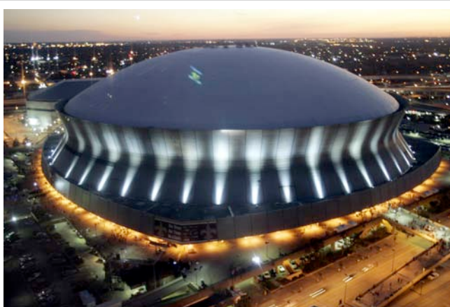
Fig. 3.6 - Louisiana Superdome, New Orleans, Louisiana
