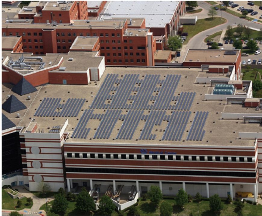
Figure 4.39: Photovoltaic system by Dallas Medical Center, Dallas SYSTEM SIZE: 337kW [ www.sunwize.com ]
