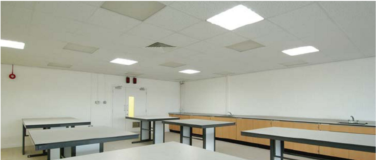
Figure 4.34 : Light diffusers [www.passivent.com]
