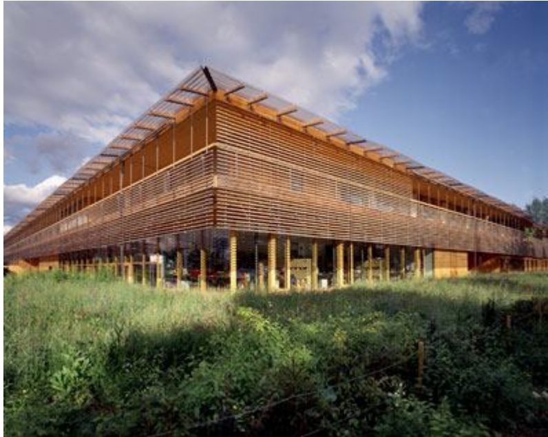
Figure 2.38 REHAB Basel Centre for Spinal Cord and Brain Injuries [archrecord.construction.com]
