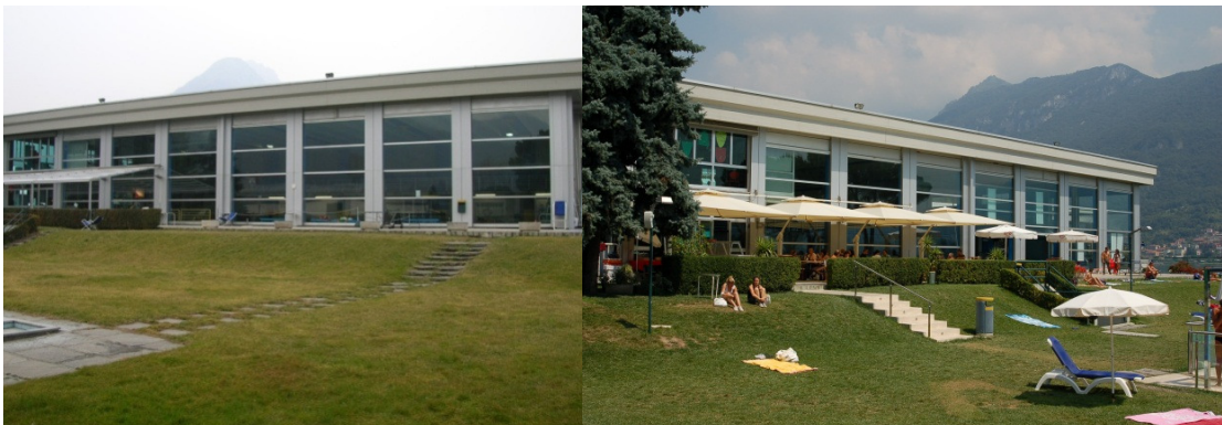
Figure 3-9 The South Façade
