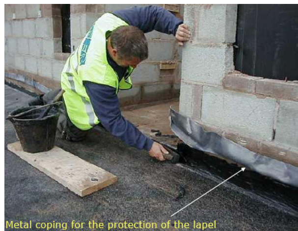
Figure 3-4 Metal Coping for the Protection of the Lapel
