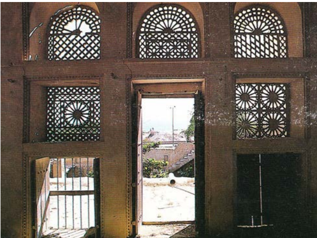
Hollow brick sun shadings
