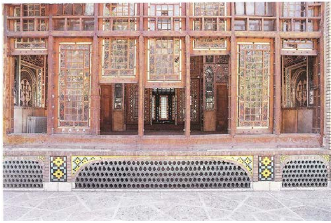
Wooden sun shading carved outer layer of the orosi windows
