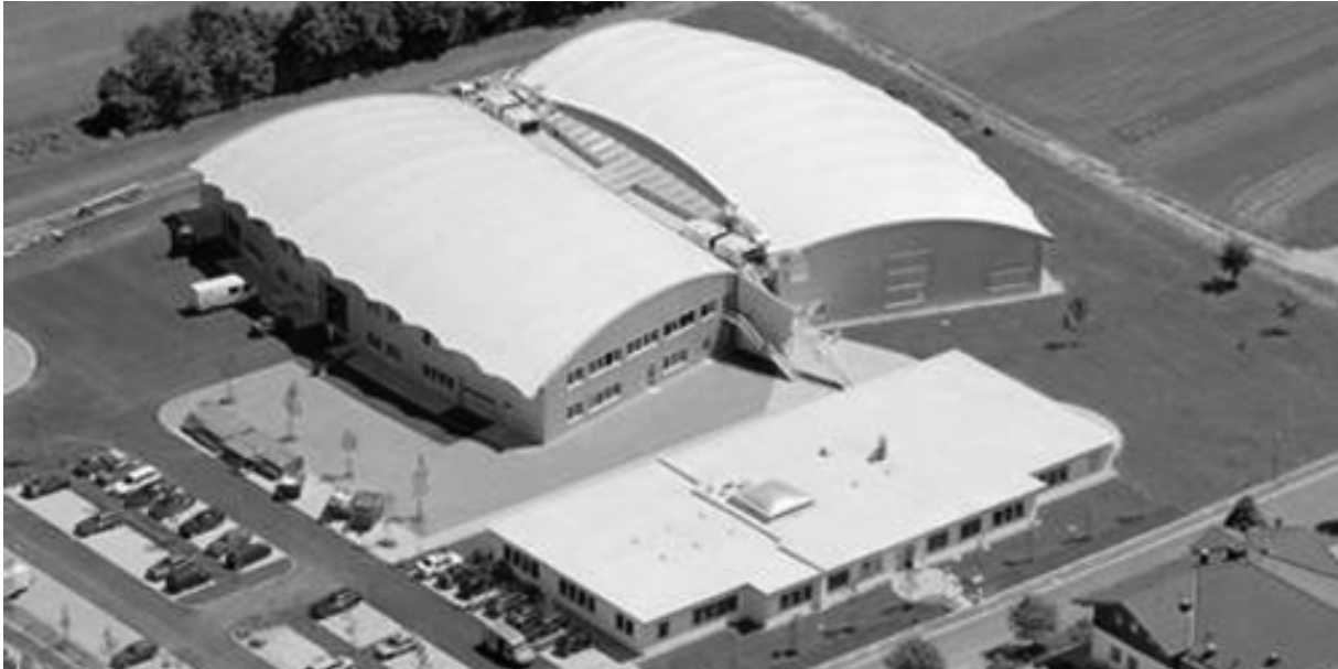
SolarNext production and administration building in Rimsting
