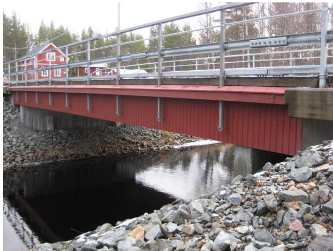
Figure 3.4 – Typical Swedish Timber bridge with glulam deck [24]
