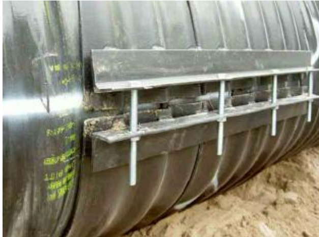
Figure 3.17 - Two pipes tighten together
