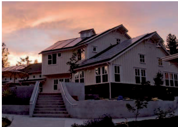
Common house-lato sud/est
