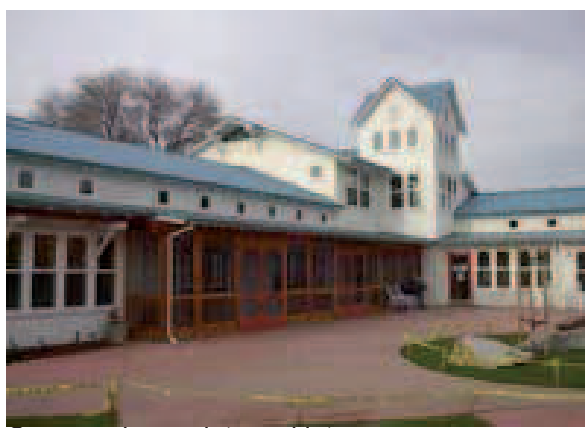
Common house-lato sud interno
