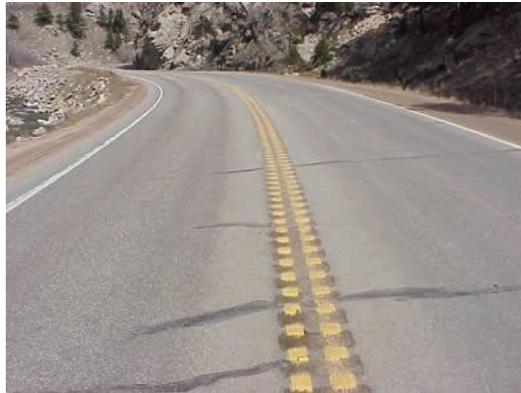
Figure 3.4: Centerline rumble strips on two-lane roadway
