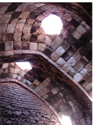
small apertures in the vaulted roof let in sufficient light
