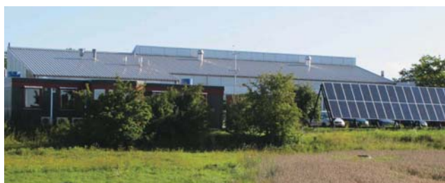
Figure 6.4 FlexHouse and PV installation at RISØ DTU
