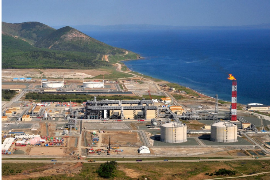
Figure 2.15: LNG plant (source: Gazprom)
