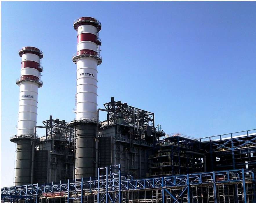
Figure 2.19: Gas turbine power plant (source: Petrom)
