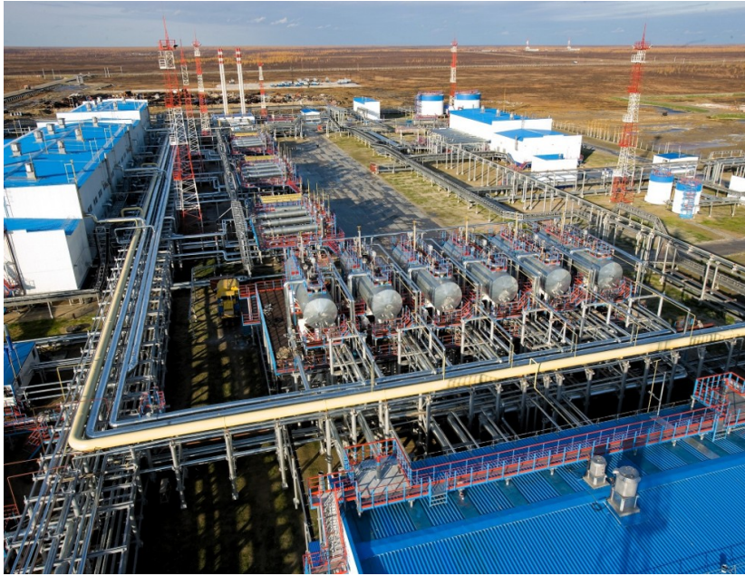
Figure 2.6: Gas treatment plant (source: Gazprom)
