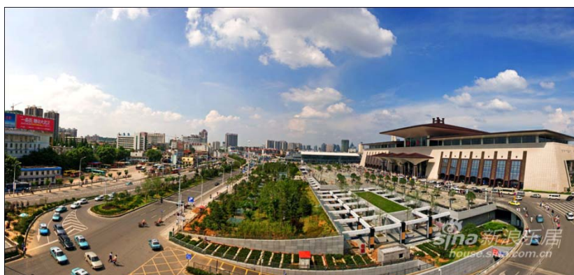
Photo 8 Wuchang Railway Station
