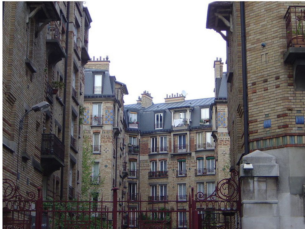
Image 2.14 HLM Housing [France] The state finances the construction of the HLM unit by low interest loans and tax-exemptions By: 2005 David Monniaux
