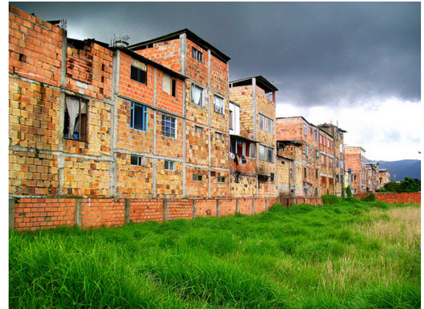
Image No. 3.14 Self-help construction traditions
