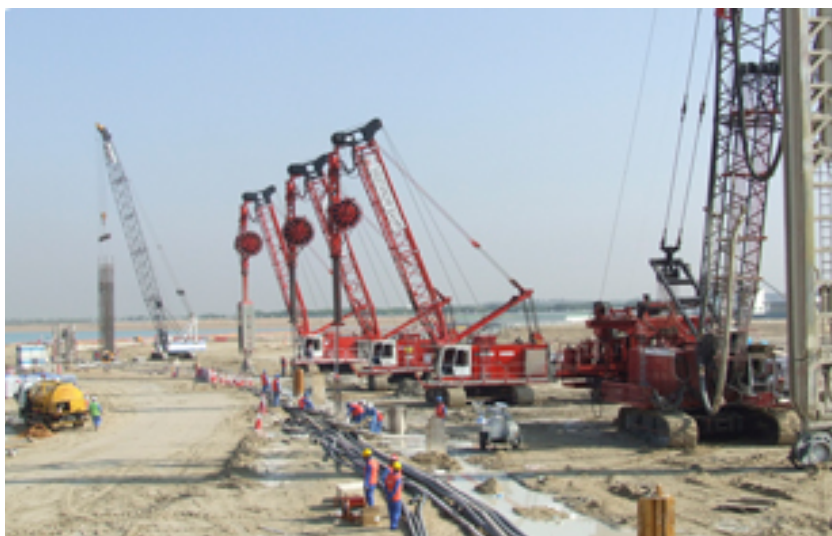
Chantier ad Abu Dhabi. AL Raha Beach
